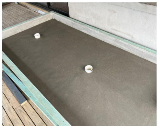
Installation of the 120SCS linear drain system (top) and the duplicate bathroom built with traditional floor wastes (bottom).
